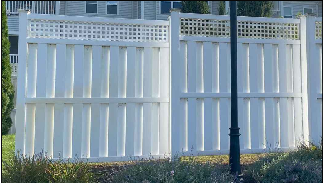
NEW SOLID SCREEN FENCE TO MATCH EXISTING SOLID SCREEN FENCE
